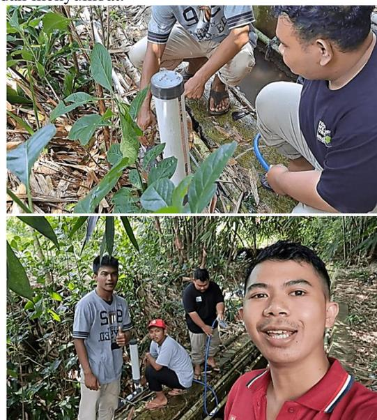
Gambar 5. instalasi pompa hydam
