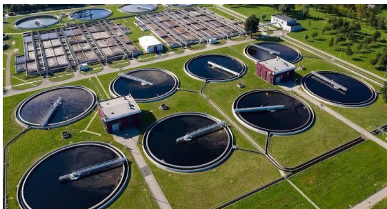
Gambar 1. Water Treatment Plant (WTP)
