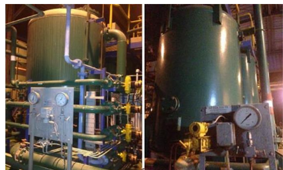
Gambar 2. Sand Filter Unit & Carbon Active Filter
