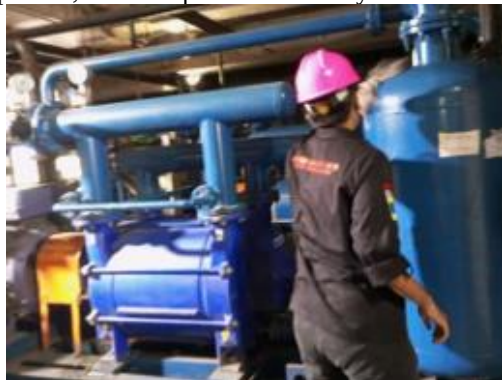
Gambar 13 Pembersihan Vacuum Pump
