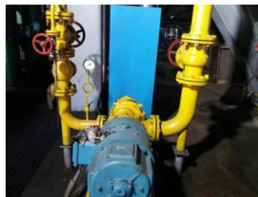
Gambar 5 DC Oil Pump
