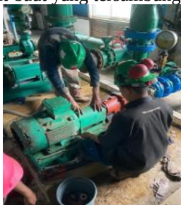
Gambar 14 Breakdown Perbaikan Feed Pump
