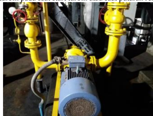
Gambar 4 AC Oil Pump
