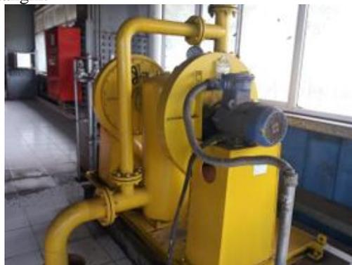
Gambar 11 *Main oil tank Exhaust Fan*
