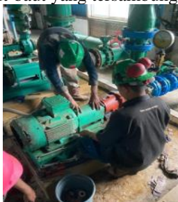
Gambar 14 Breakdown Perbaikan Feed Pump
