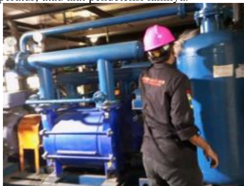
Gambar 13 Pembersihan Vacuum Pump
