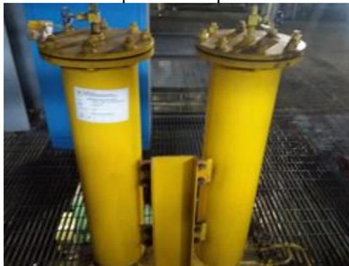
Gambar 8 Turbine Lube Oil Conditioner
