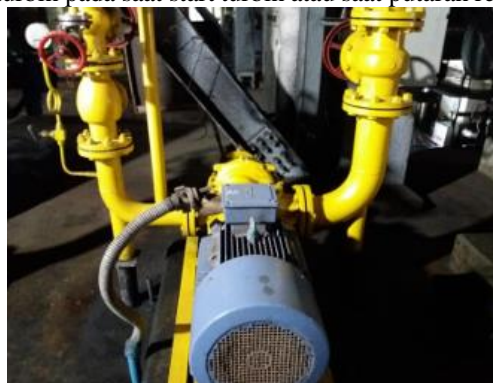
Gambar 4 AC Oil Pump
