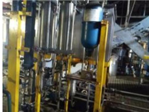
Gambar 10 DEH (*Digital Electro Hydraulic*)
