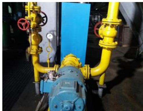
Gambar 5 DC Oil Pump
