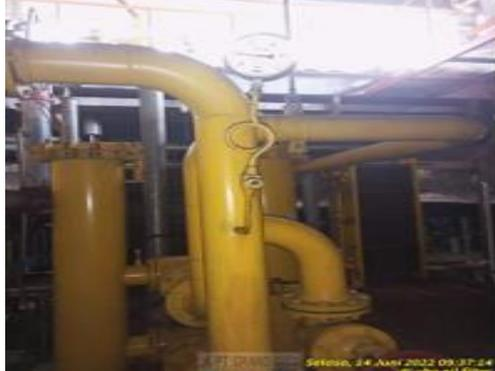
Gambar 7 Lube Oil Filter
