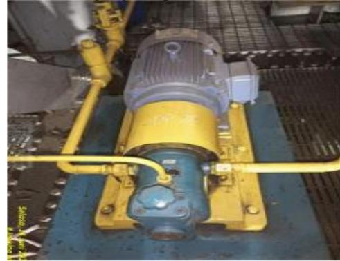
Gambar 9 Jacking Oil Pump
