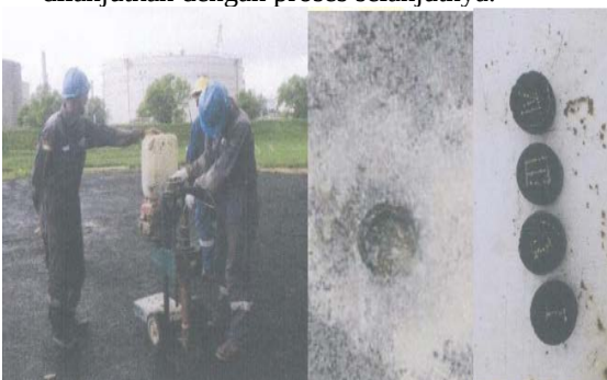
Gambar 5. Proses Core drilling Test
