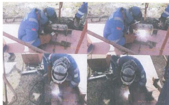
Gambar 7. Proses pengelasan annular
