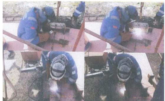
Gambar 7. Proses pengelasan annular
