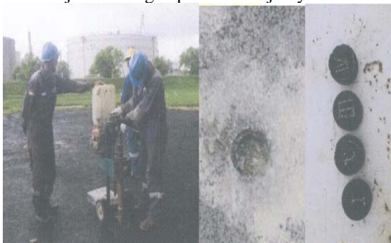
Gambar 5. Proses Core drilling Test
